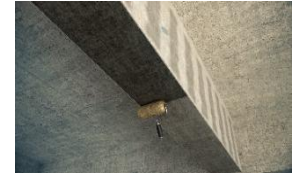
Applying epoxy resin adhesive
