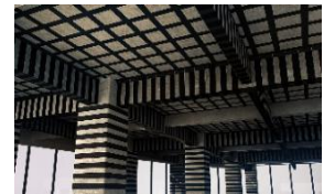
Curing and protecting
